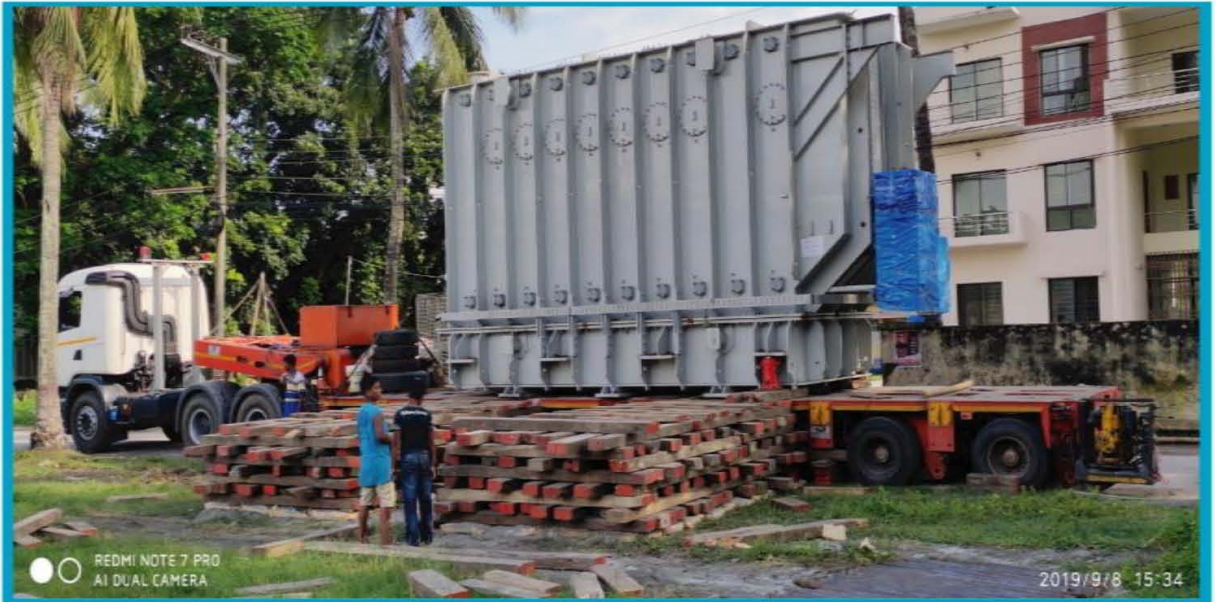
NESCO(Northern Electricity Supply Company Ltd. 195 ton Energypac
