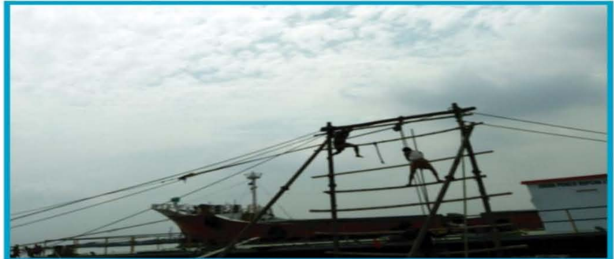
Temporary Jetty Construction
