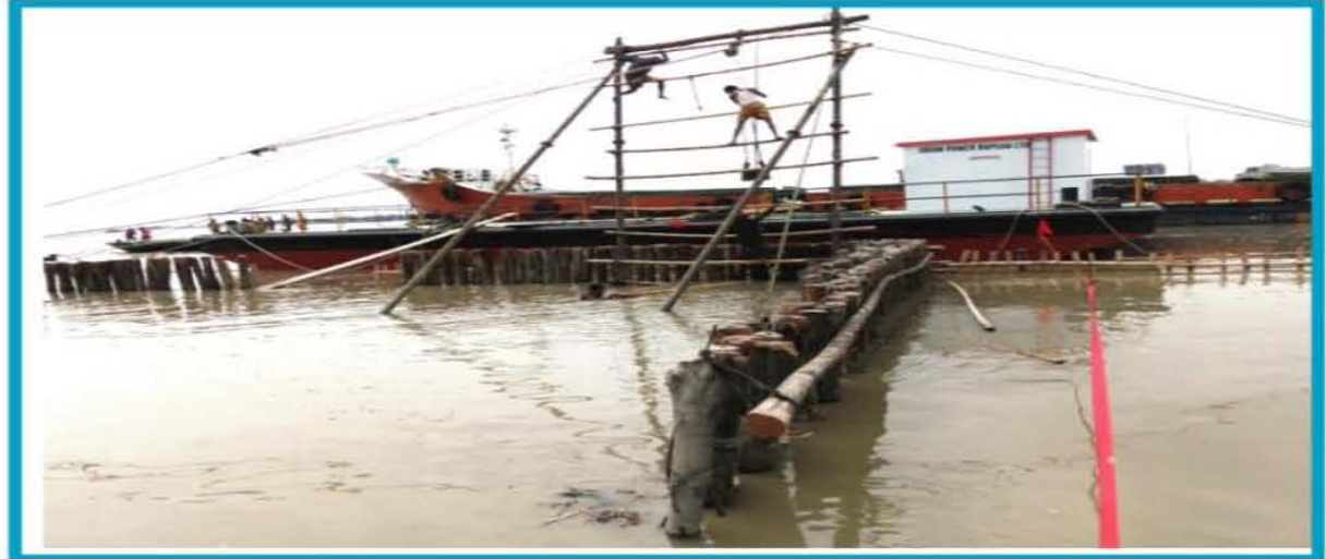
Temporary Jetty Construction
