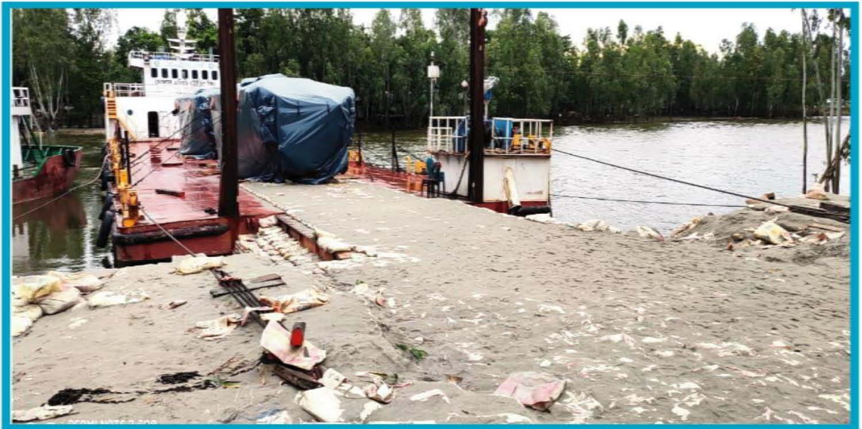
Thakurgoan Power project Gauripur 162 ton MAN Energy solutions
