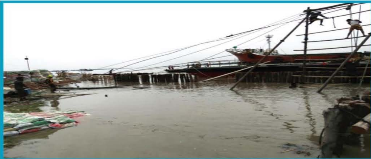
Temporary Jetty Construction
